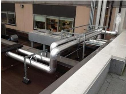
Exterior aluminum cladding on heat trace insulation
