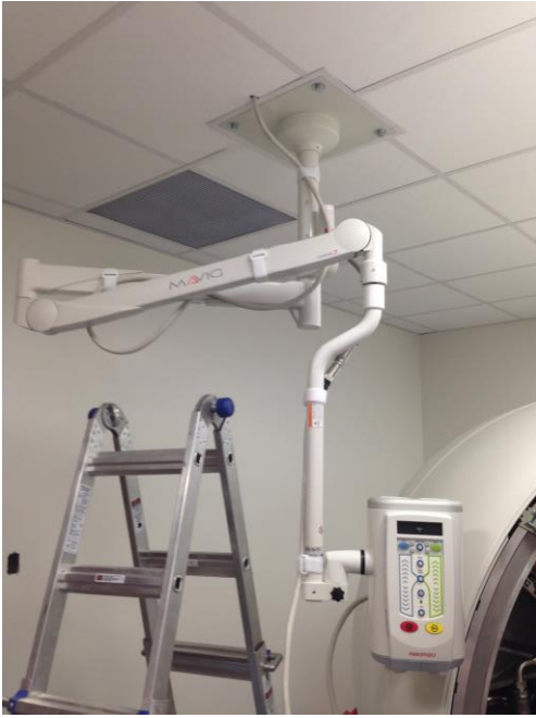
Injector installed.
